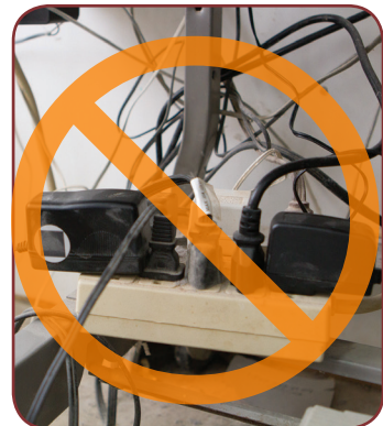
Overloaded Electrical Socket
