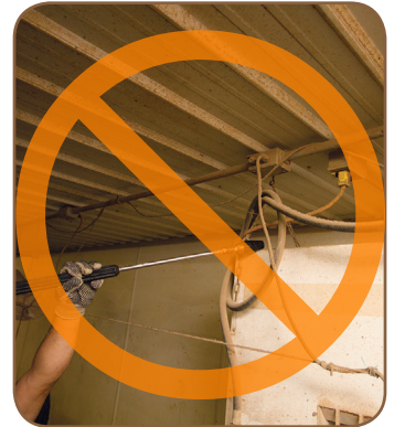
Aiming power washer toward electrical outlet
