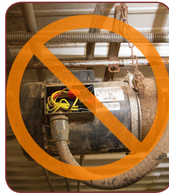
Exposed wires
