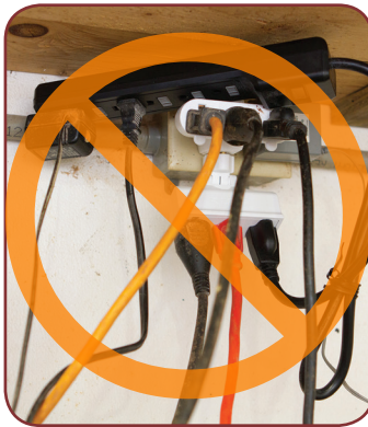
Overloaded socket
